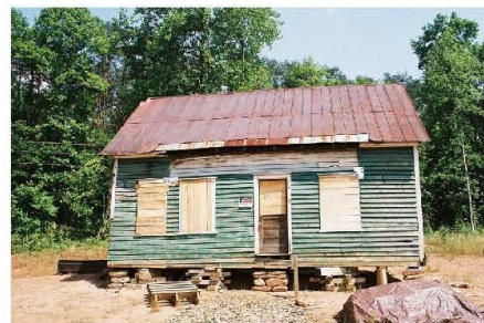
This photo shows the slave cabin resting on the original rock piers in its new home at the Nacoochee Valley African American Heritage Site & Nature Preserve. Stone mason David Vandiver will reassemble the rock chimney and hearth. Photo by Jeanne Cyriaque
