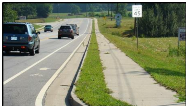
Figure 7. Bike Lanes and Sidewalks along GA Hwy 75
